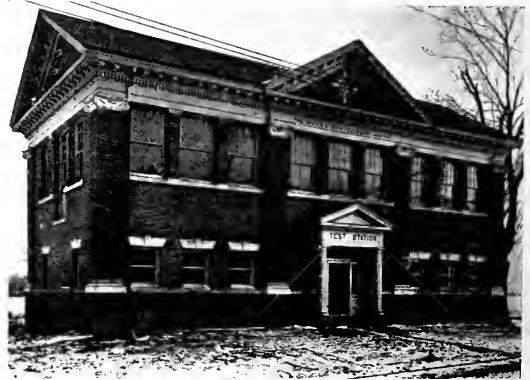
FIG. 17.—REPEATER AND SWITCHING STATION, THOMPSON'S CORNERS, O.
